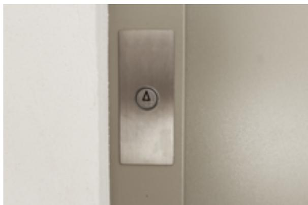
External keypad, button with braille system and backlit.
