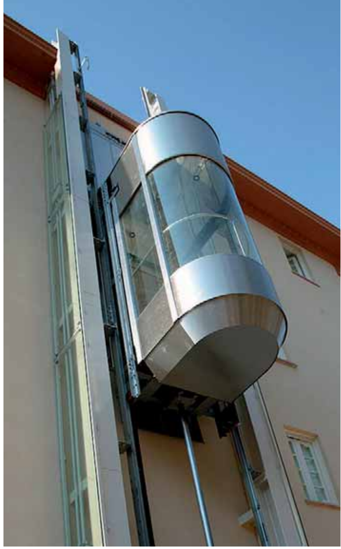
Vivienda particular_ Ascensor con cabina semicircular recta a hueco. Private house _ Lift with semicircular car straight to shaft.
